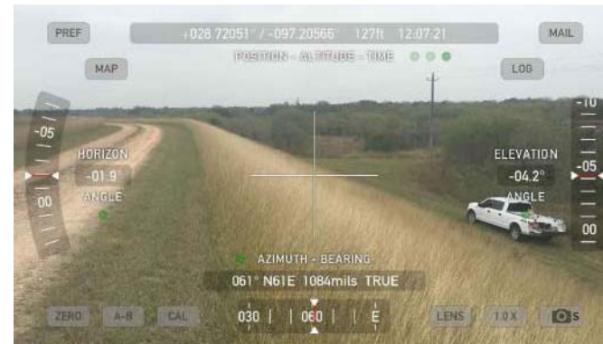
2109 - Top of Levee / Exterior
