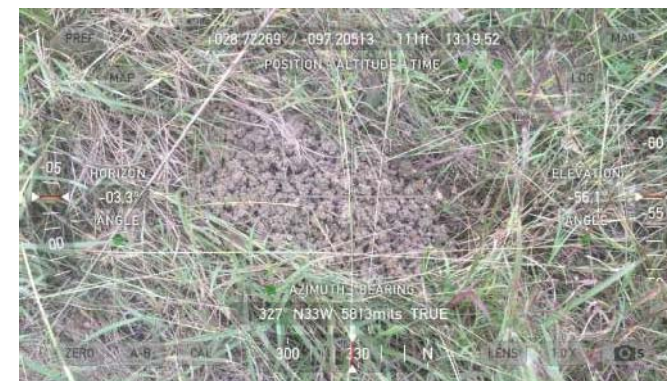
2153 - Exterior Toe (Rodent Grubbing)
