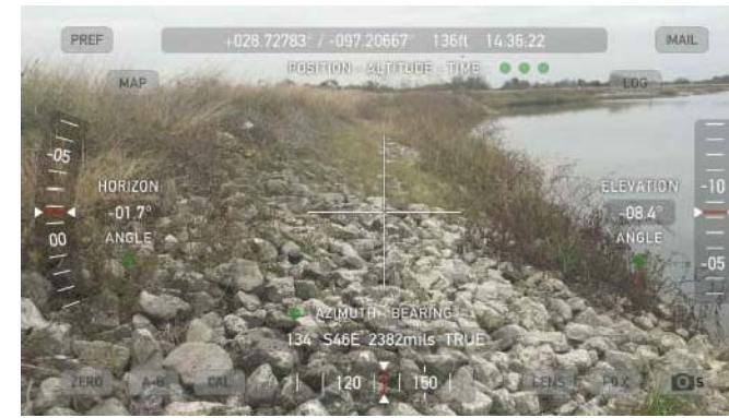
2221 - Interior Slope Protection
