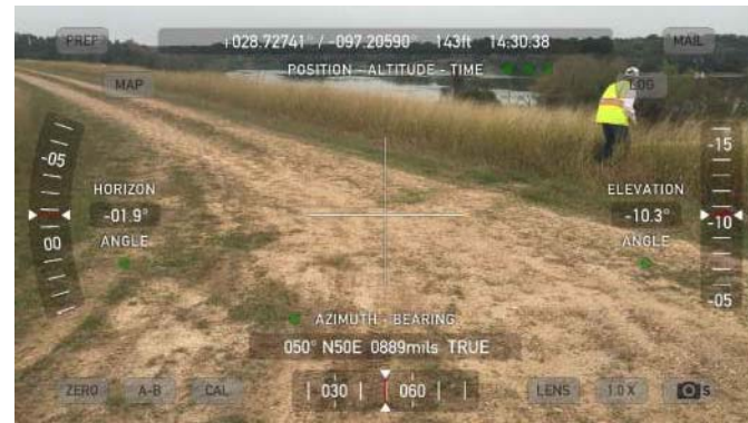
2209 - Top of Levee, Seep Collection Discharge Pipe (shallow burial)
