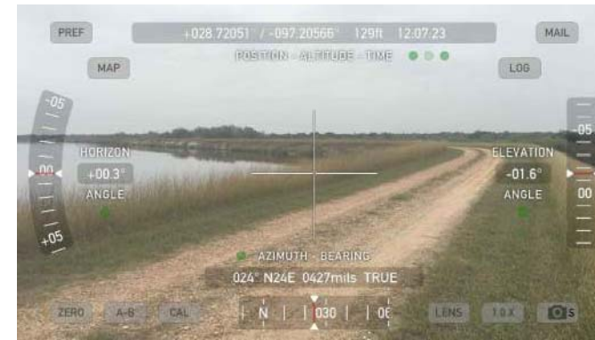
2110 - Top of Levee / Interior Armor
