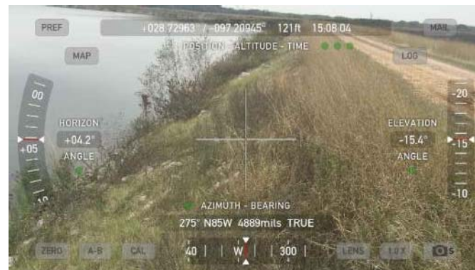
2304 - Interior, Slope Protection (Stone) Covered by Grass
