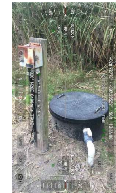
2179 - Seepage Collection System Sump
