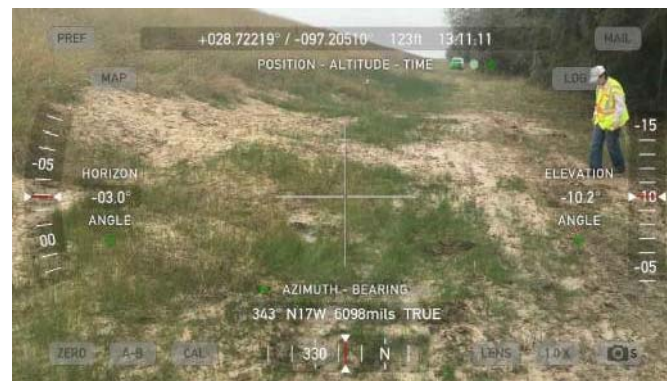
2148 - Exterior (Wet Area)
