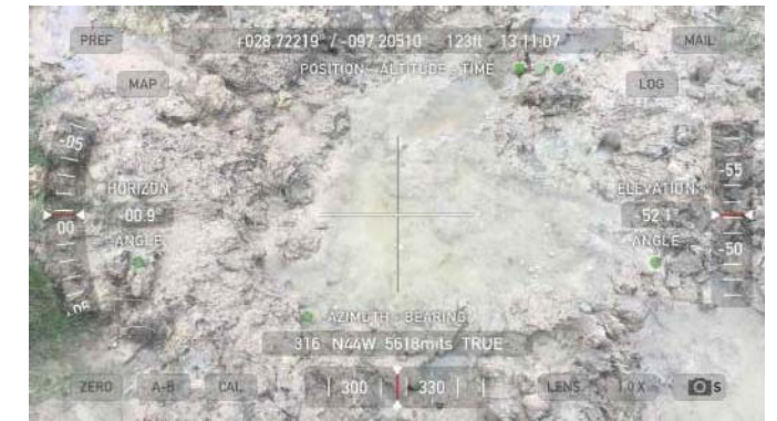
2147 - Exterior Toe (Wet Area)
