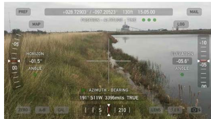
2300 - Interior / Bank Erosion
