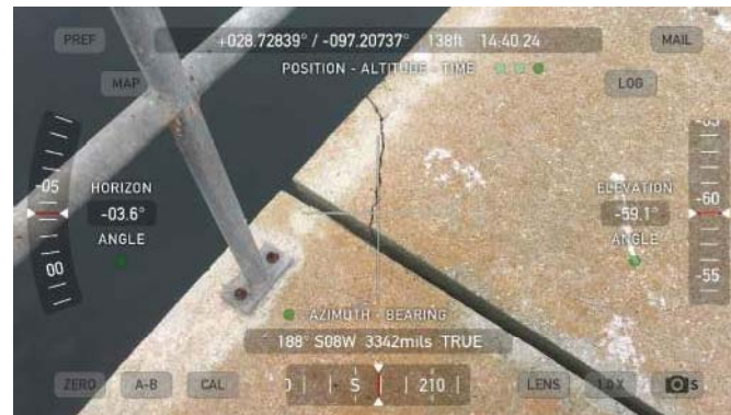
2230 - Concrete Decking Joint (at first bent)
