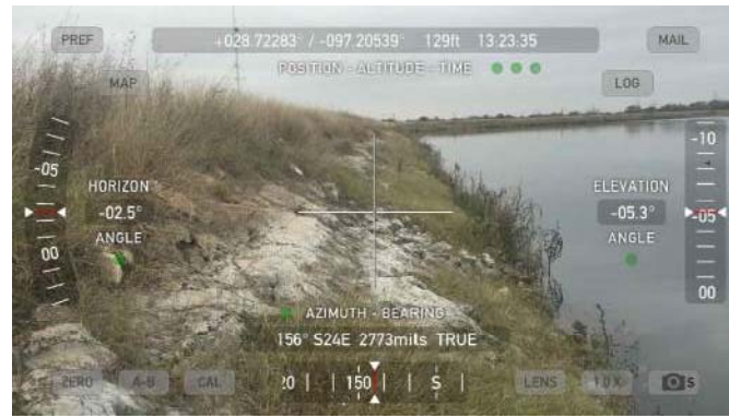
2159 - Interior Slope Protection
